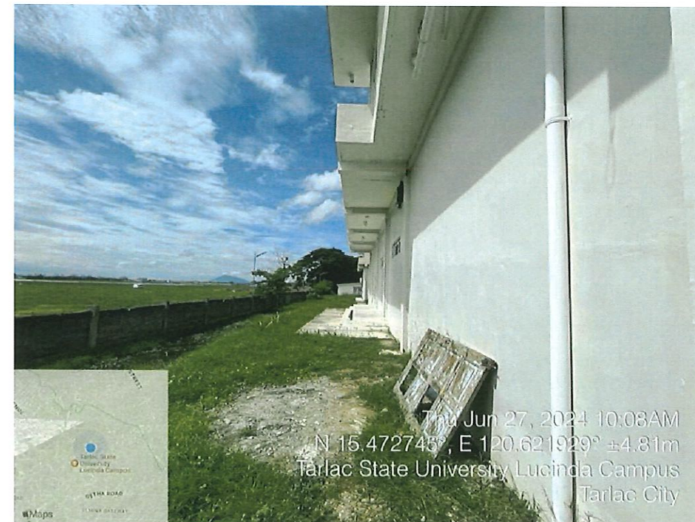
REAR OF THE BUILDING
