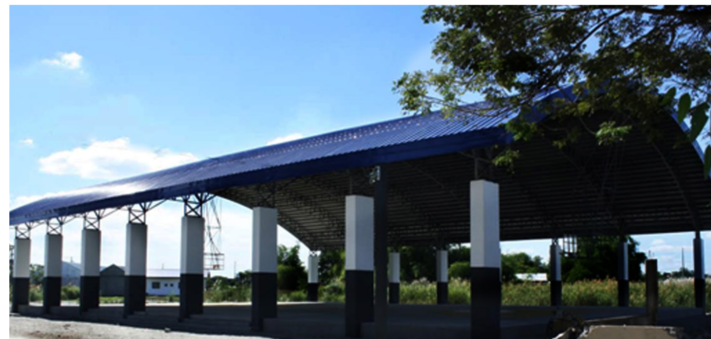
Repair of TSU Gymnasium Roofing
